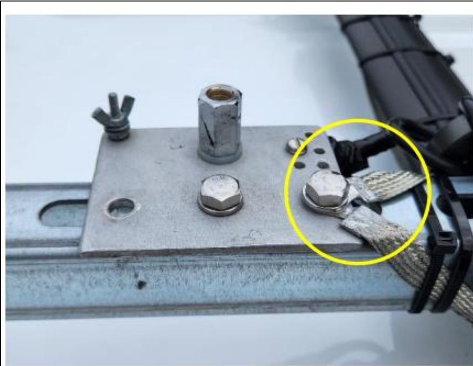
Aluminum Mounting Plate with 1/2" Bonding Straps
